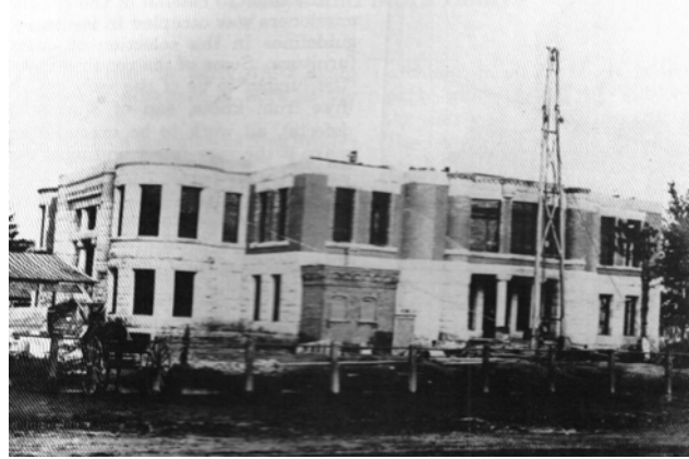
Courthouse 1889 (in progress)
